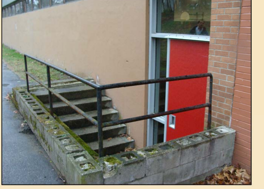
STAIRS AT NORTH GYM
